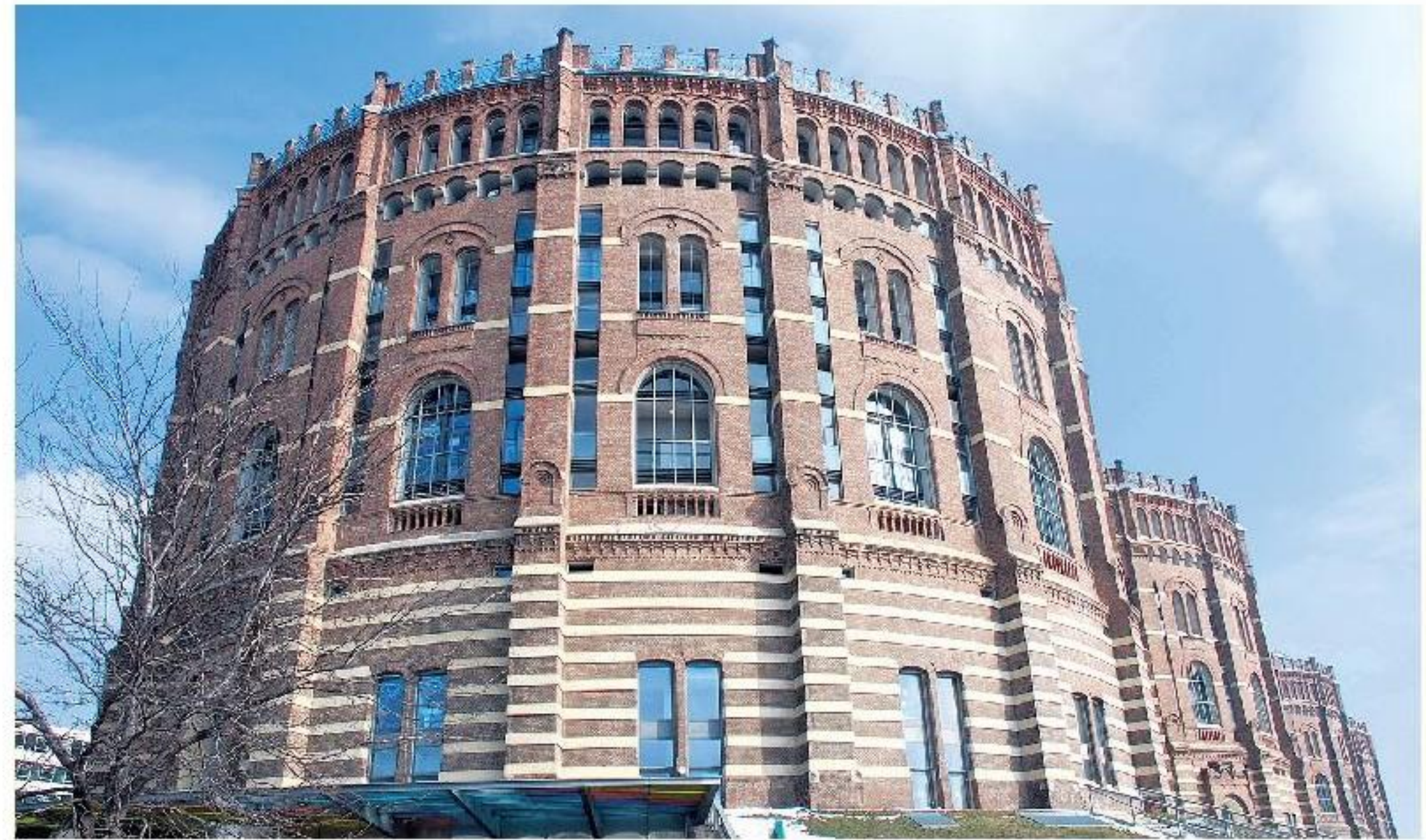
Each Gasometer building is 65 metres wide with individual interior designs Photo: Duncan Smith
