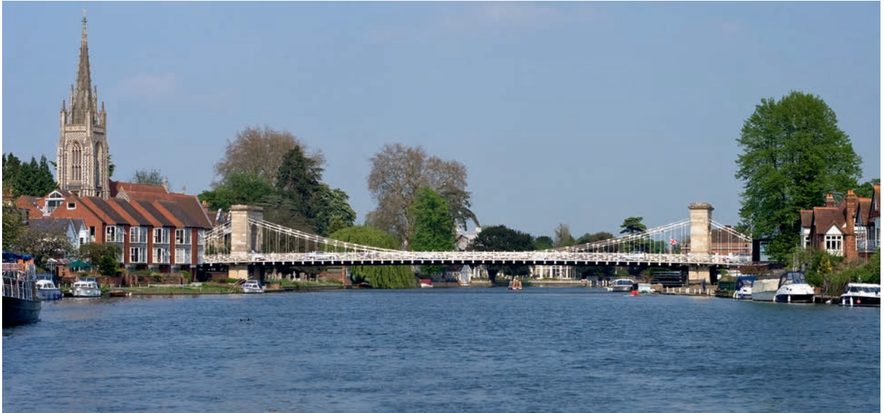
Marlow Suspension Bridge gracefully spans the River Thames. It opened in 1832 (photo © Andrew Chambers / dreamstime.com).
